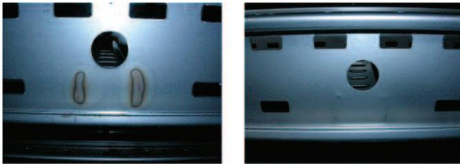
Fig. 12. Detailed shot of annealing colours that have been removed by water blasting.
