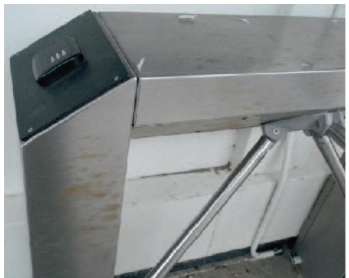
Fig. 11. Turnstile manufactured from stainless steel 316 that has been attacked by aerosols.
