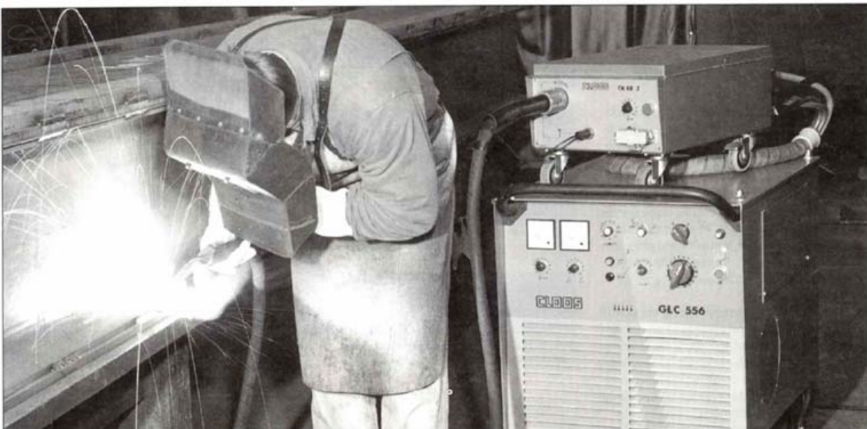
GTAW welding of a stainless steel tube
