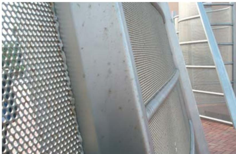
Picture 4. Rust pits showing on the design's posts.
