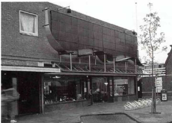
Awning shop – Alphen a/d Rijn – The Netherlands. The corrugated parts are of stainless steel
