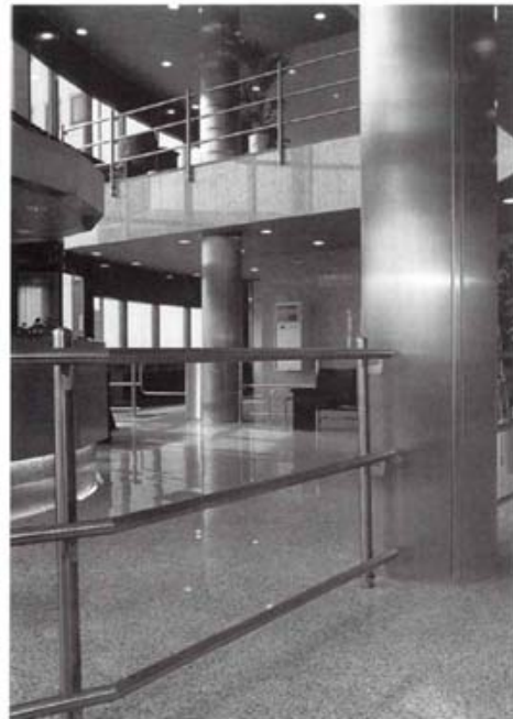
Europagebouw – Haarlem – The Netherlands Two stainless steel sheets are covering two concrete pillars
