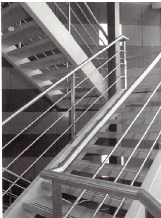
Banisters of stainless steel. The balusters exist out of two fixed flat bars welded at the inside.
