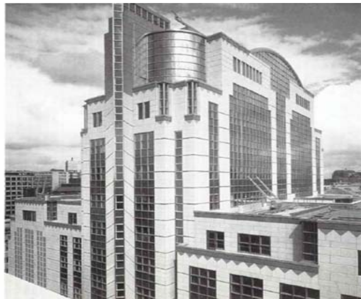
One American Square Tower, London. In this project stainless steel is used as curtain wall at the top of the building (AISI 316), for the fixing of the granite (AISI 304) and the snap-in-construction (AISI 316)
